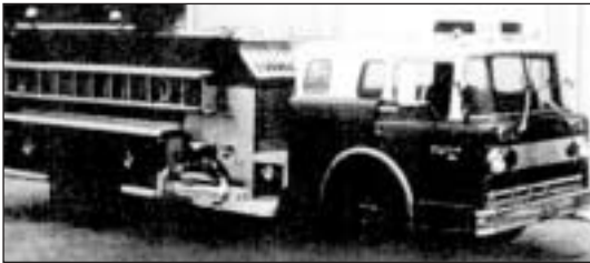
1983 Ford C Series 5 Man Cab Diesel / Automatic 1000 GPM Pump & 750 Tank
